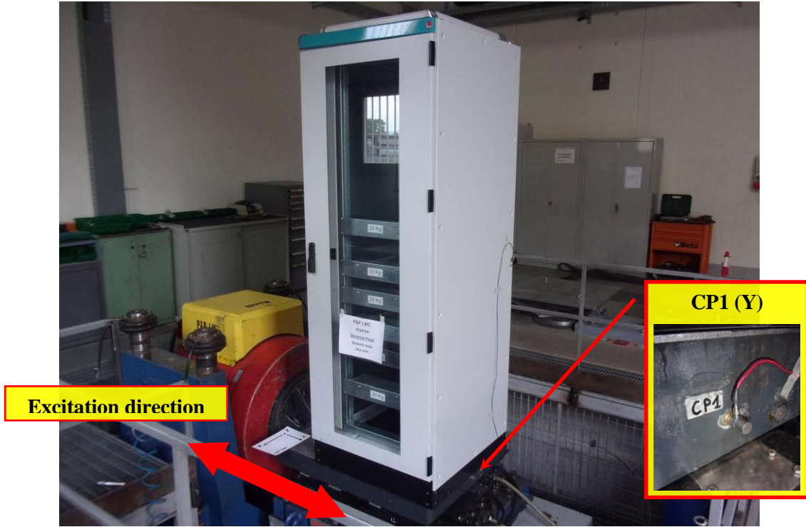
Photo 3: Test configuration for seismic test in Y direction
