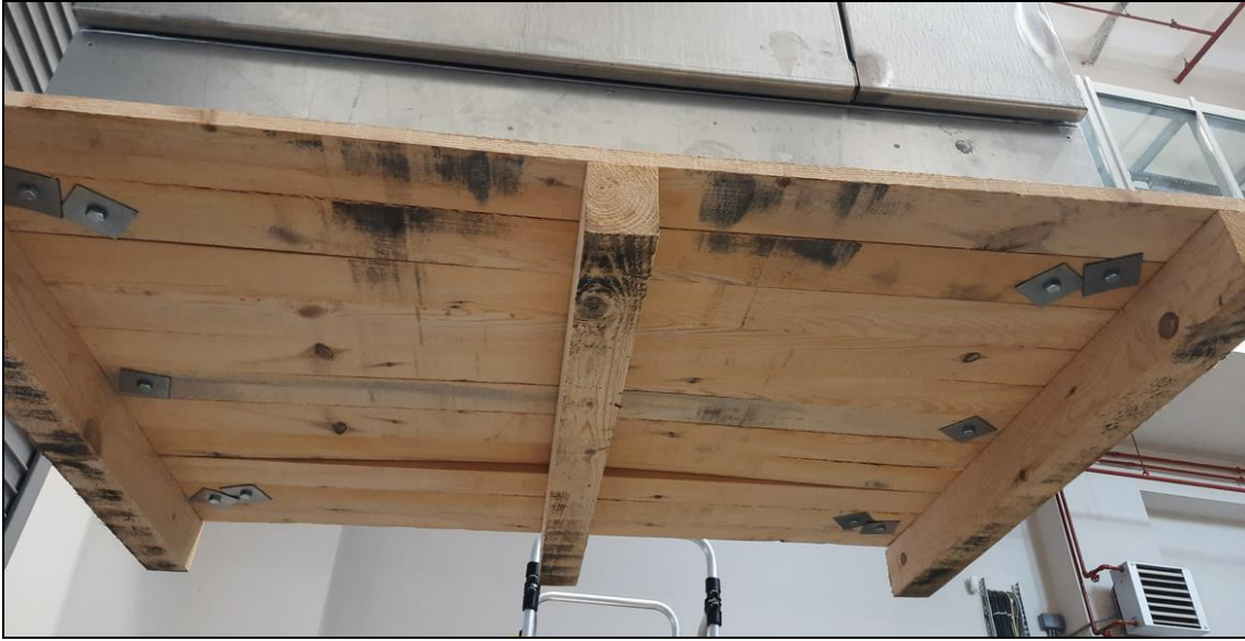
Picture 4. Transport Pallet Connection Details
